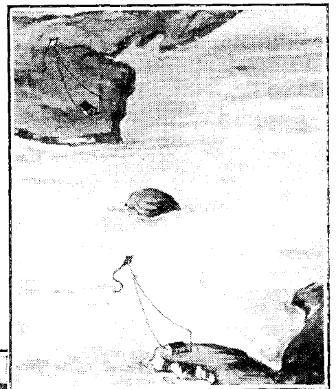
Elevated cylindrical aerials were first used at the Needles station, Isle of Wight. Kite aerials were also experimented with.
